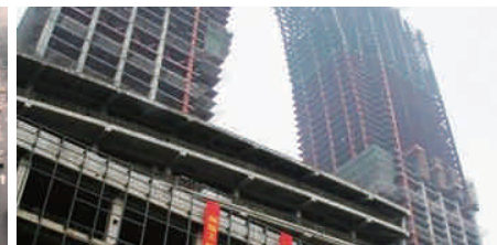
苏州东方之门施工 Gate of the Orient,Suzhou Construction Site
