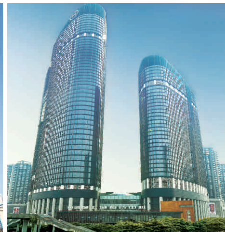
重庆第一高楼 Tallest Building in Chongqing
