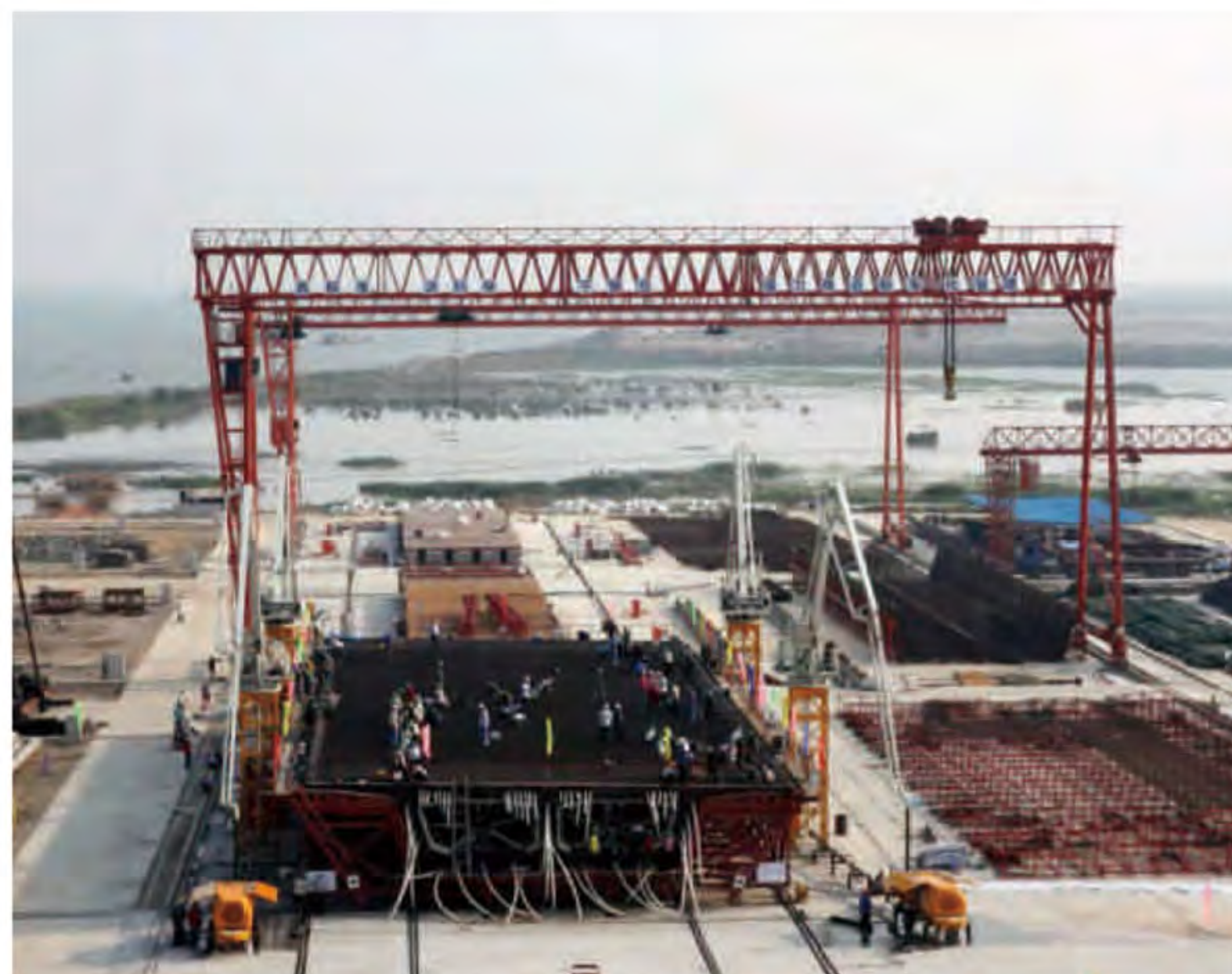
江苏苏通长江大桥施工现场 Jiangsu Sutong Changjiang Highway Bridge Construction Site
