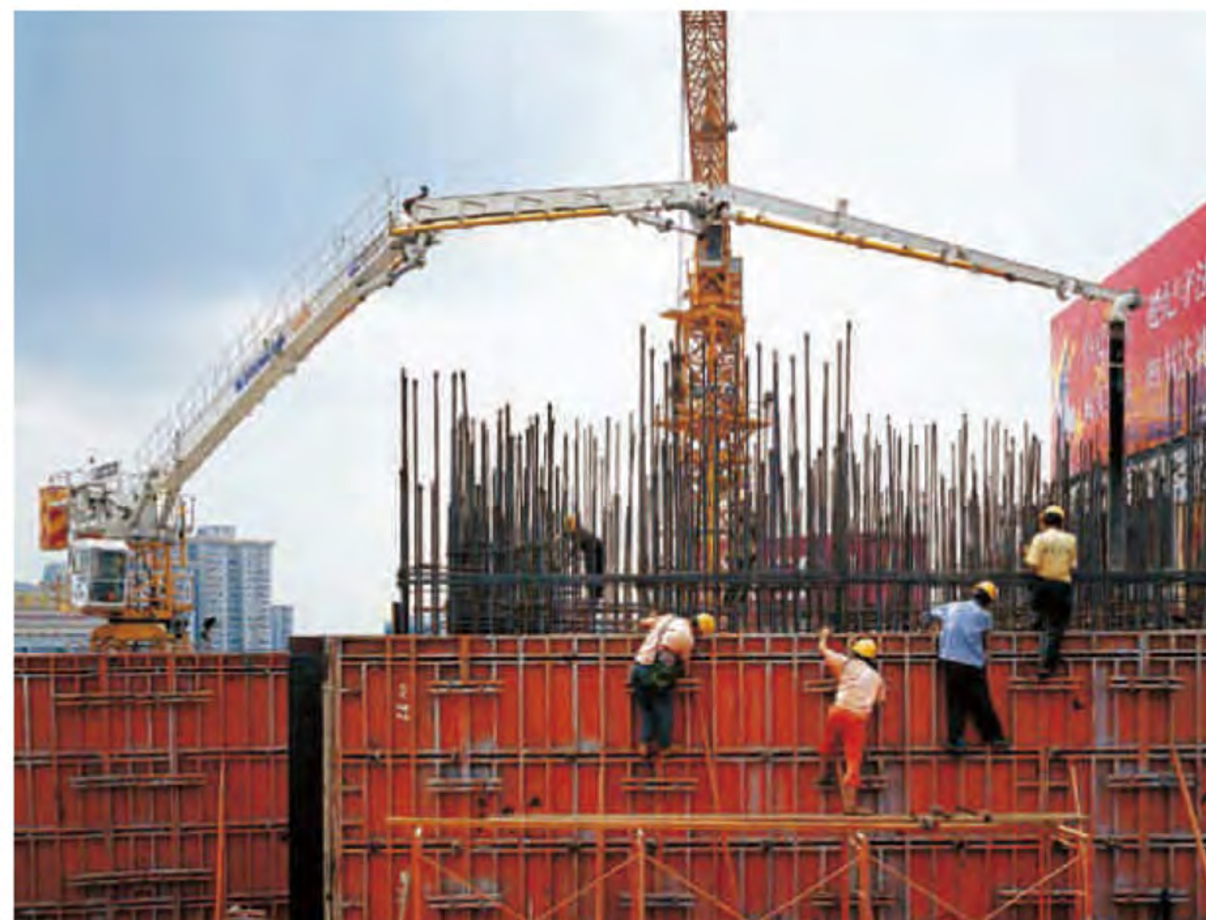
广州天河城东塔写字楼施工现场 Construction Site of Guangzhou Tianhe City Oce Building East Tower
