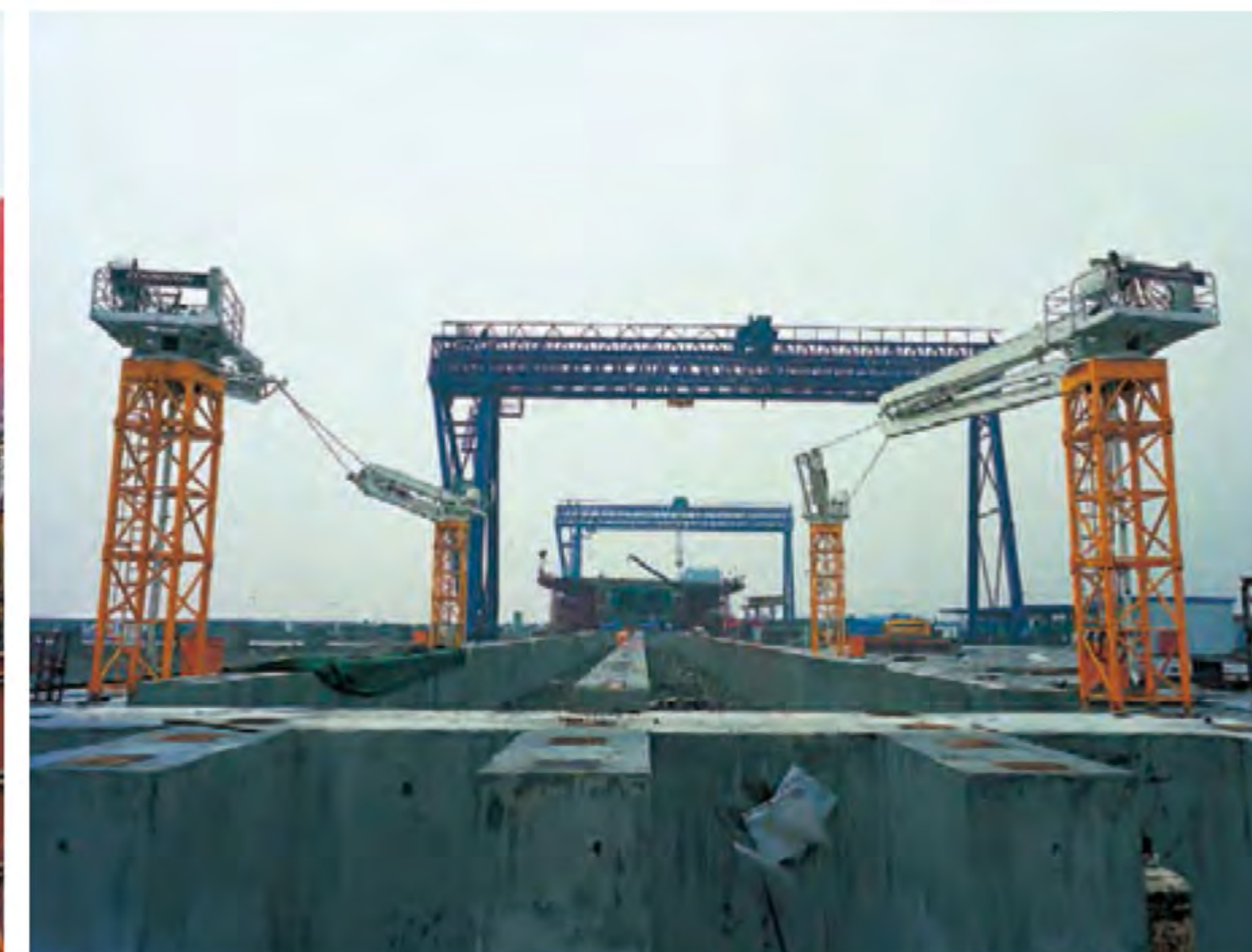
杭州湾大桥施工现场 Hangzhou Bay Bridge Construction Site
